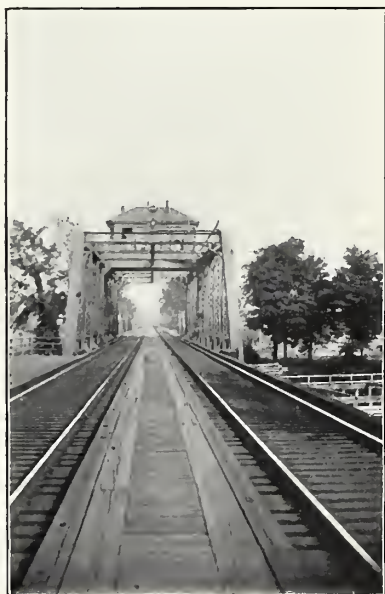
ERIE RAILROAD BRIDGE, LOOKING EAST.
